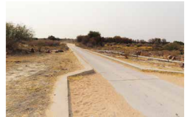
Photo: Annika Hoffmann, Witvlei Bridge, 2024
