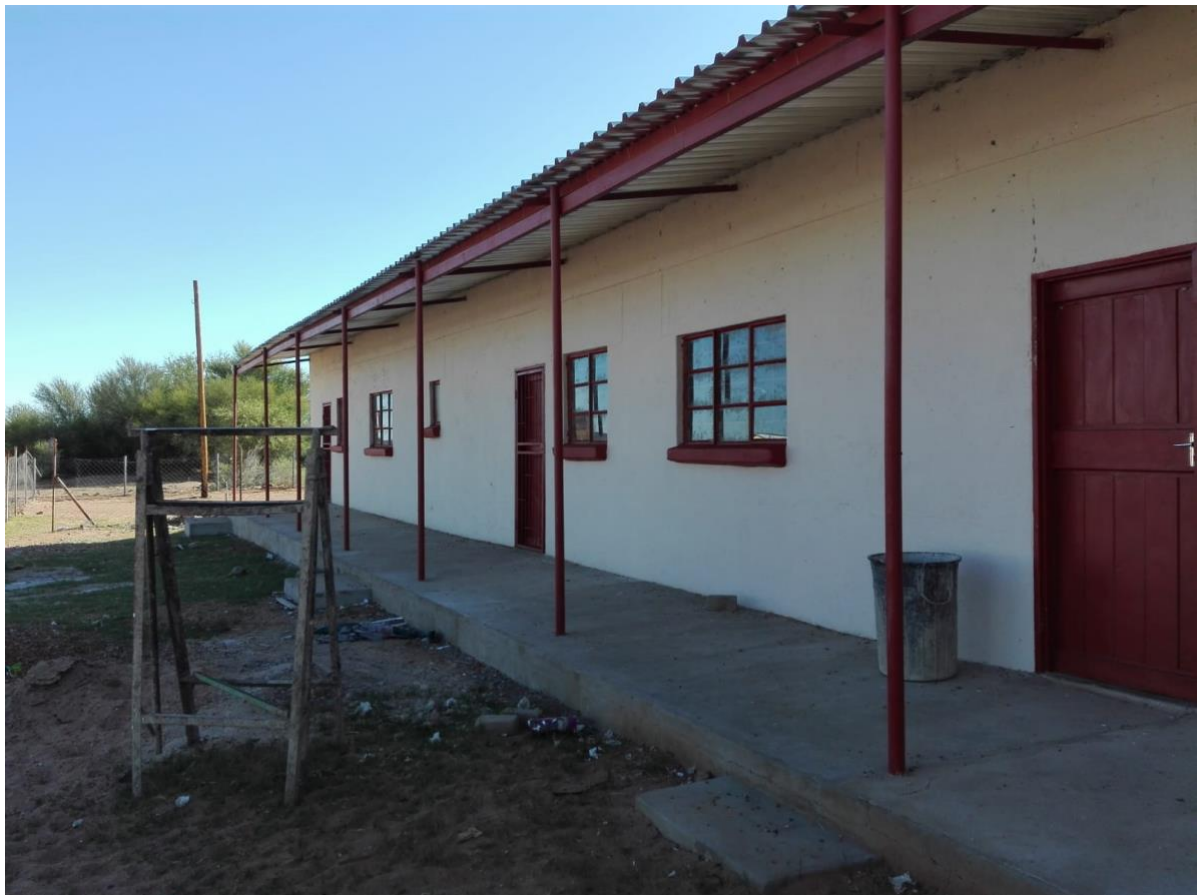
Bau neuer Klassenräume an der Nossob Combined School, Witvlei
